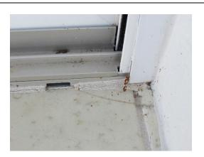
Spalled stucco & concrete on unit 433
