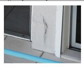
Typical aged & failing sealants unit 444
