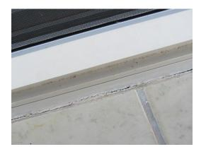
Typical aged & failing sealants unit 444
